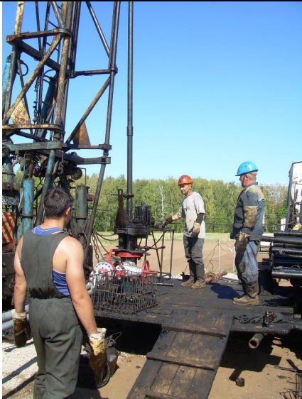
Photo 4. The moment of the cassette FCR lowering into the injection well as a part of PCP suspension
