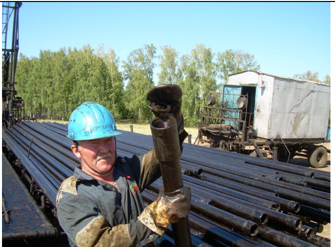
Photo 2. Filling the stopper ring into the sleeve of PCP
